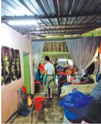
Damages caused by flood
