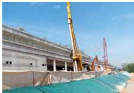
Slope protection and silt fence
