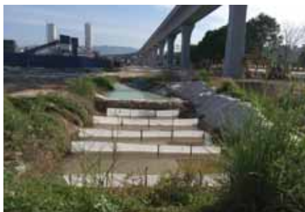
Check Dams &amp; sediment filtration fence
